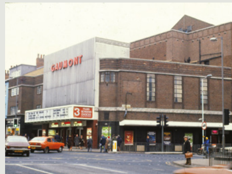
The Gaumont with the cladding installed in 1968. It was renamed Odeon in January 1987, closed in April 2008, and demolished in 2009. (Photograph by Allen Eyles.)
